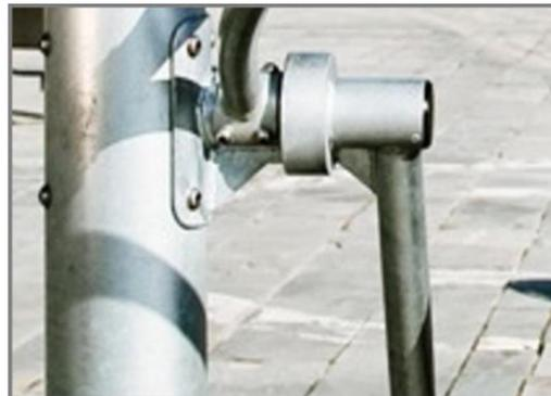
Handlebar and pendulum arm are made of a hot-dip galvanized steel tube 1.9" with a wall thickness of 0.13". A strong connection which is necessary to withstand the forces created during this movement.
