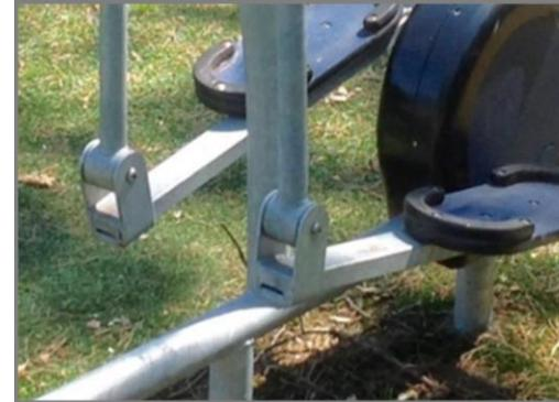
The frame and moving steel parts are constructed of hot-dip galvanized steel tube's 2.37" x 0.13", 1.5" x 0.16" and squared tube 2.36" x 1.18" x 0.12". All moving connections have a stainless steel AISI 304 shaft and two ball bearings.
