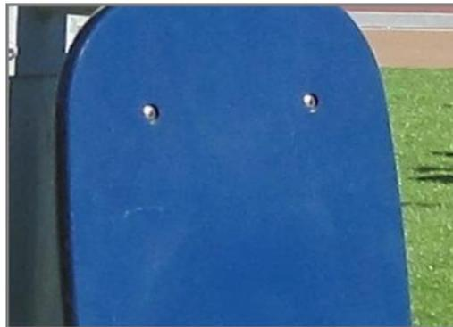
Panels are constructed of 0.75" machined EcoCore™. EcoCore™ is a highly durable, ecofriendly material, which is not only recyclable after use, but also consists of a core produced from 100% recycled material
